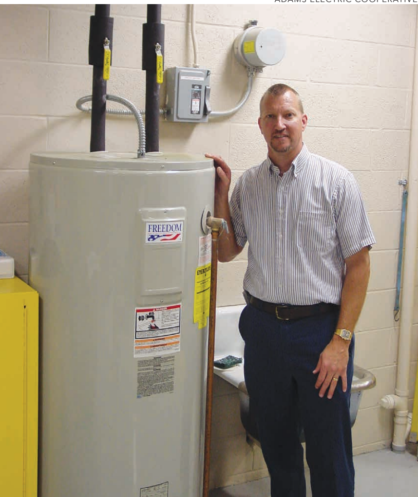
A SWITCH THAT SAVES: Brian Shearer, senior staff engineer at Gettysburg-based Adams Electric Cooperative, stands beside a water heater equipped with a load control receiver. When members volunteer to have these systems installed in their homes, it helps the cooperative manage purchased power costs and offer stable rates.
