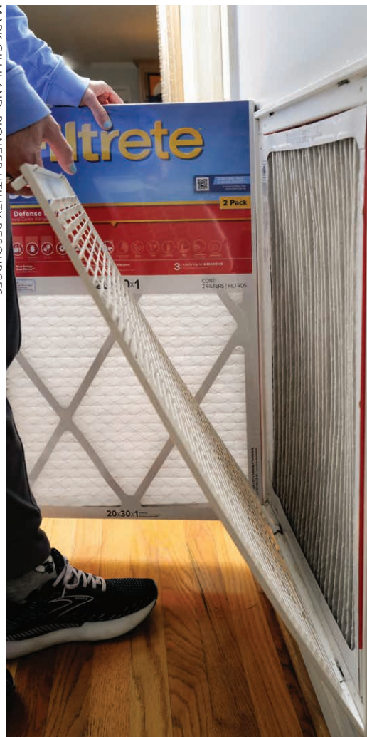
FILTER FIX: Replacing your furnace filter is a low-cost and easy way to protect your equipment and maximize efficiency.
